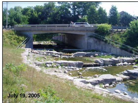
Left Photo: Pre-construction view of fish barrier (gabion basket) located on Harmony Creek (Branch 3) below Harmony Road.
